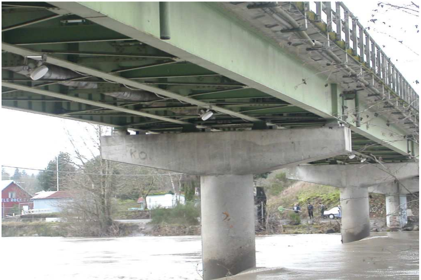
Figure 1: Microwave surface velocity sensors installed on the Cowlitz River bridge at Castle Rock, WA. The white antennas in the figure are four of the eight sensors that were installed on the bridge at various distances across the river.
