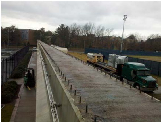
Figure 5. Guideway before installation
