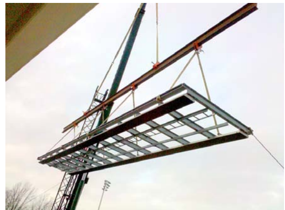
Figure 4. Crane lifting stator and rail module
