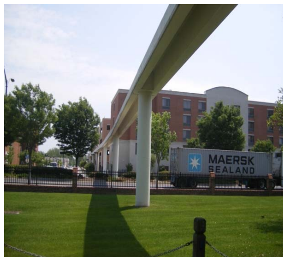
Figure 2. Existing ODU guideway
