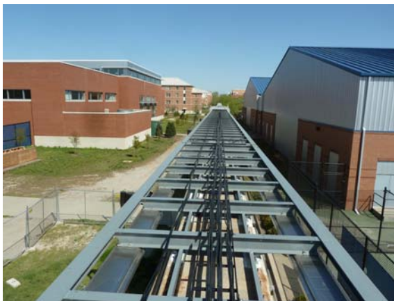
Figure 6. Guideway after installation
