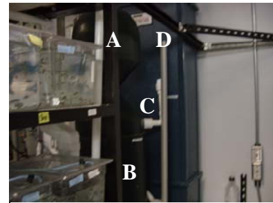
Figure 6.7 A) Biofilter B) Biofilter drain valve C) Air purge plug D) Degassing tower
